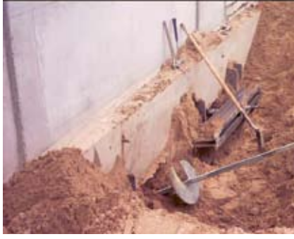
Torealign beam, 38 CHANCE® helical tieback anchors were installed between Atlas Resistance® piers.
