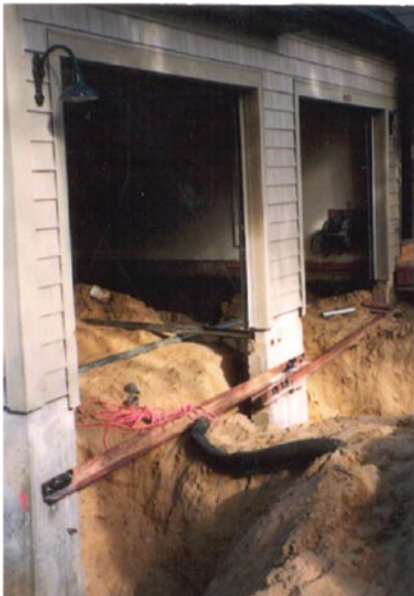
Above, side of the garage showing installed piers No. 1, 2, 3 and 4.
