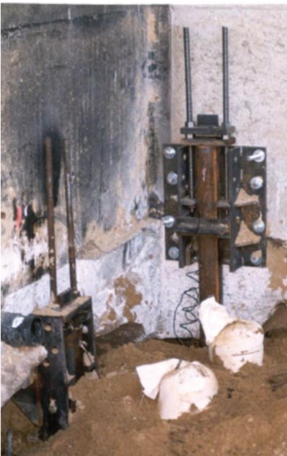
Below, an Atlas Resistance® Standard Continuous Lift Pier and a Continuous Lift Plate Pier are shown fully installed, with the load transferred to the pier and with the magnesium anodes attached.
