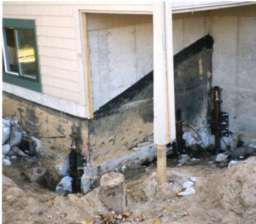
Piers 7, 8, 9 and 10 at the rear of the house near the garage during the lift. Notice the 25-ton hydraulic rams installed on each pier.
